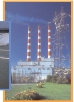
EMR-3706 Natural gas-powered electrical generating station, Nova Scotia
