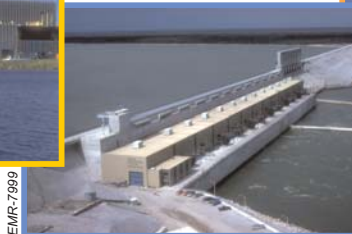
EMR-7999 Hydroelectric dam, Manitoba
