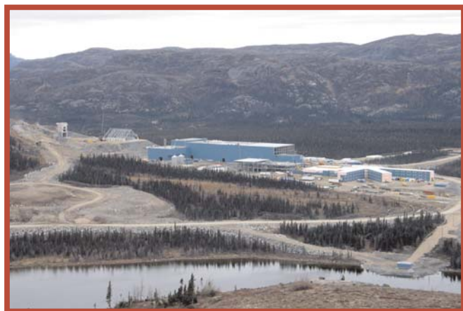
Concentrator building and accommodations, Voisey's Bay, NL, October 2004
