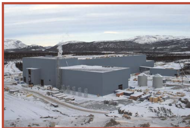
Concentrator building, Voisey's Bay, NL, November 2004
