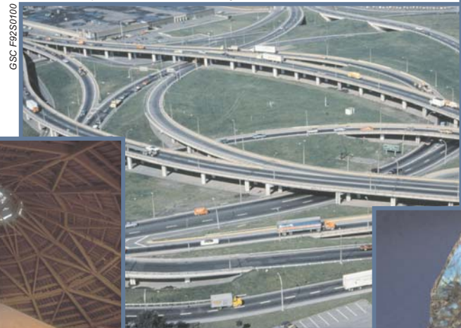
Décarie-Metropolitan Boulevard interchange, Montreal, Quebec
