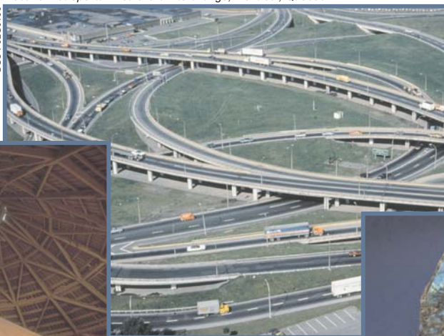
Décarie-Metropolitan Boulevard interchange, Montreal, Quebec
